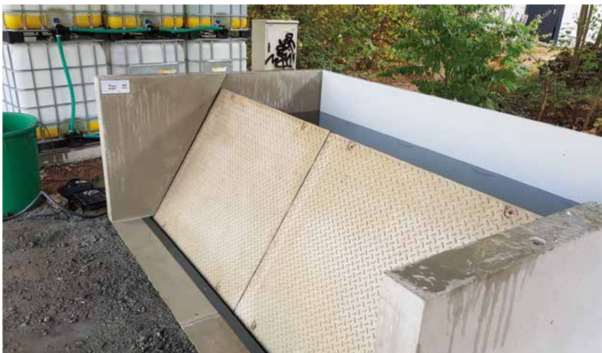
Fig. 9: "Real-life" functioning of the flood barrier after water accumulation
